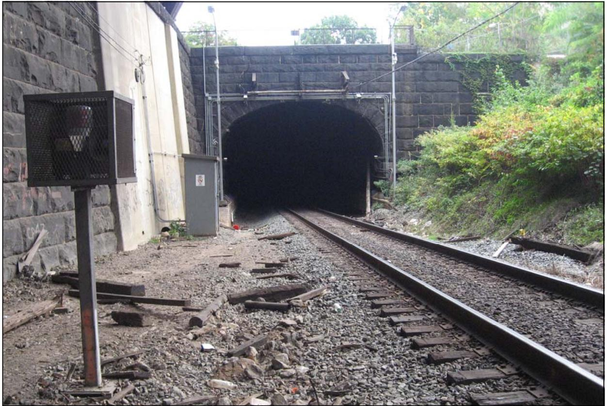
**The existing single-track, low-clearance Virginia Avenue Tunnel (looking east toward Maryland), constructed in 1904, is a choke-point for rail freight movement through the Washington region.**
